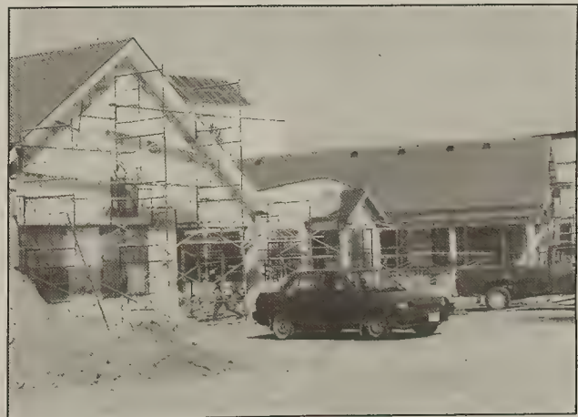
Carleton's new day-care centre under construction.
